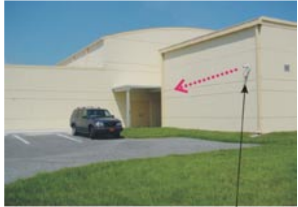
ELECTRONIC SURVEILLANCE SYSTEM STRATEGICALLY PLACED TO MONITOR BLIND CORNER AT PERIMETER OF SCHOOL BUILDING
