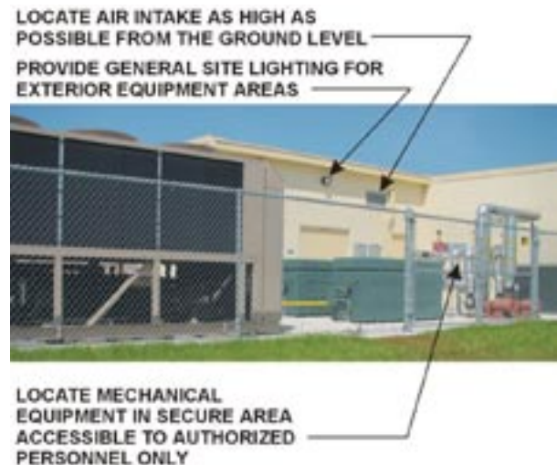
Figure 4.2.1 HVAC/Mechanical Equipment Example
