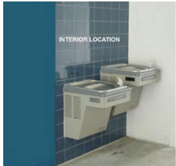
Figure 4.3.1 Typical Wall-hung Type Fixture
