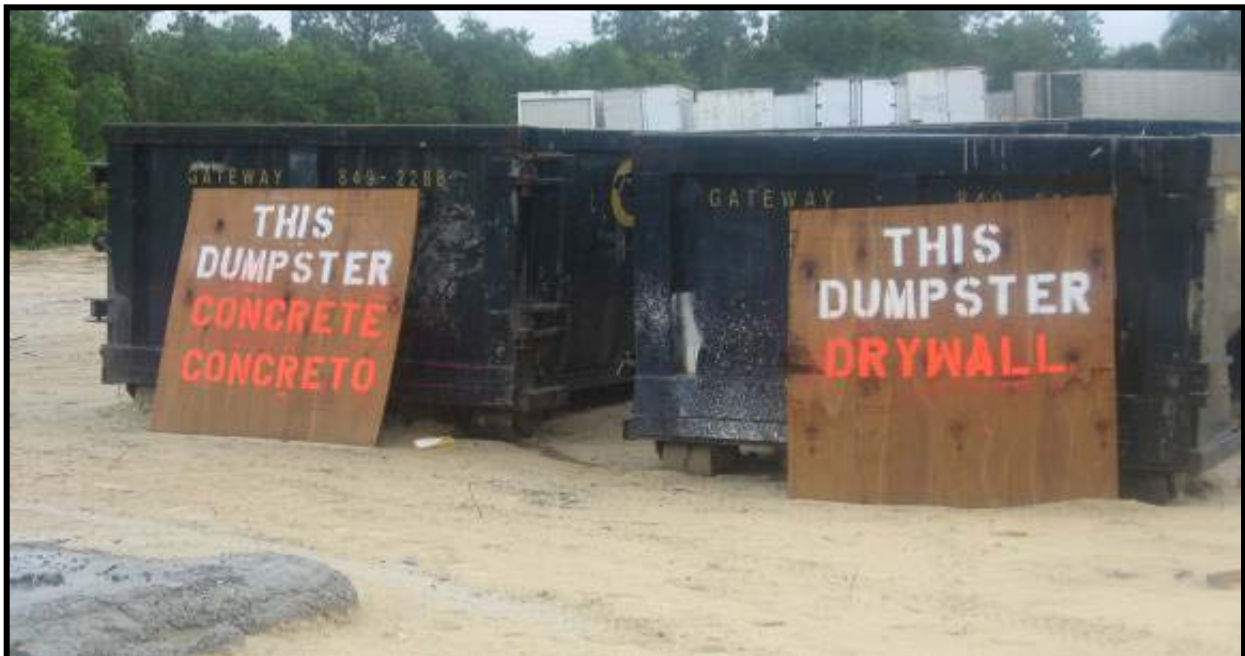
Figure 6.5 Separate dumpsters were used to facilitate the recycling of materials used on the project.
