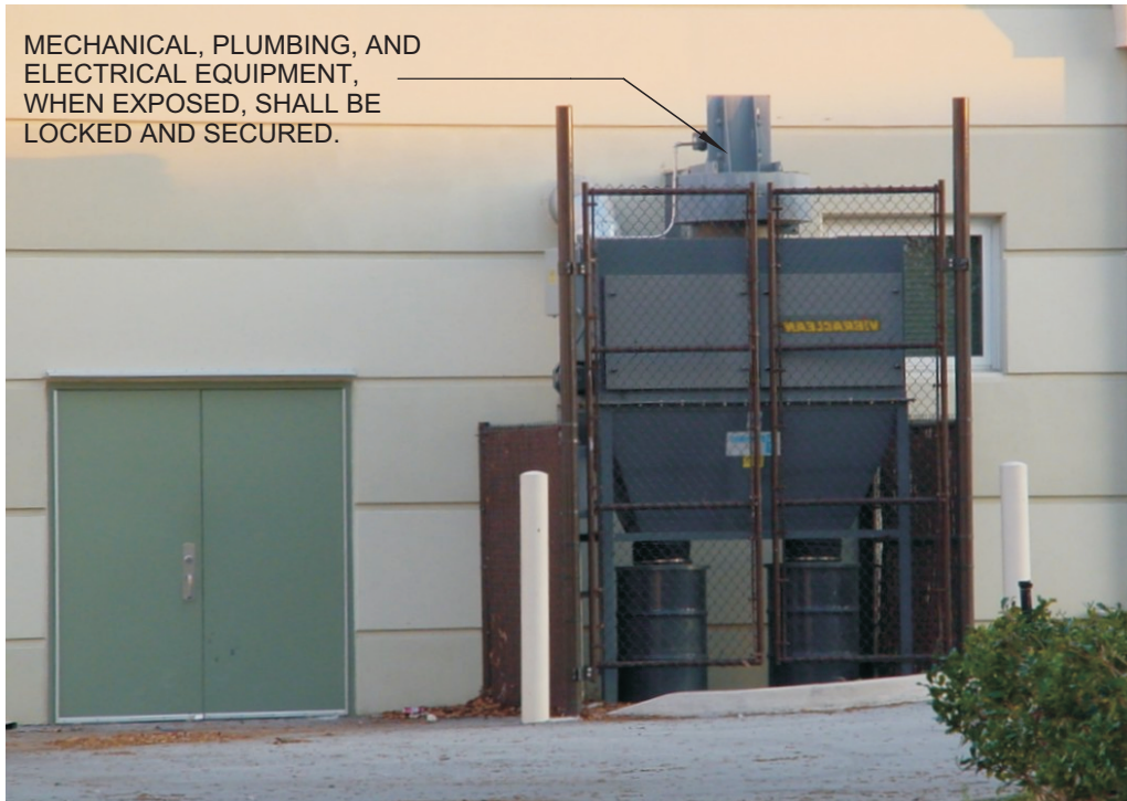
(f) Required fenced equipment
