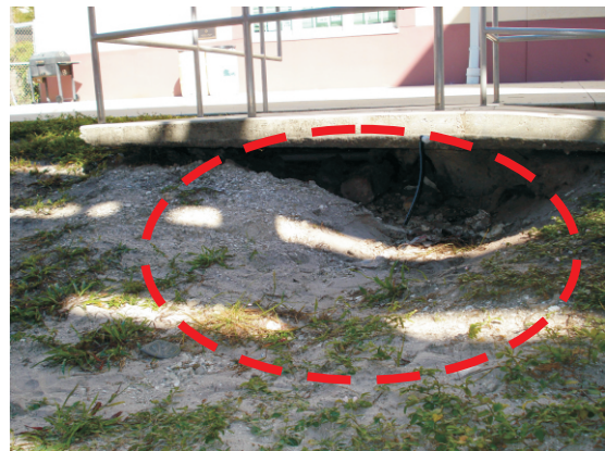
(b) Hazardous Site Conditions - Washouts around Buildings
