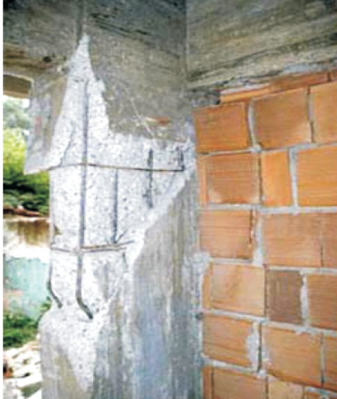
(a) Material Hazard - Spalling concrete with exposed rebar
