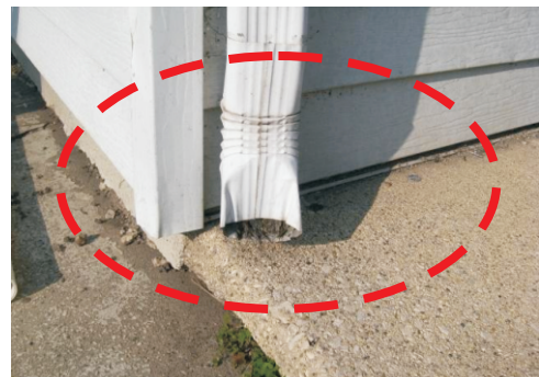
(c) Downspouts, gutters and roof drains should be maintained in good condition.
