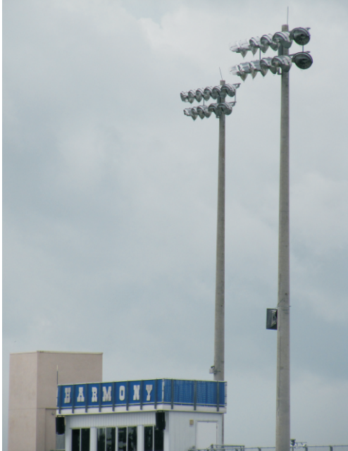
(a) Example sports field lighting with light shields
