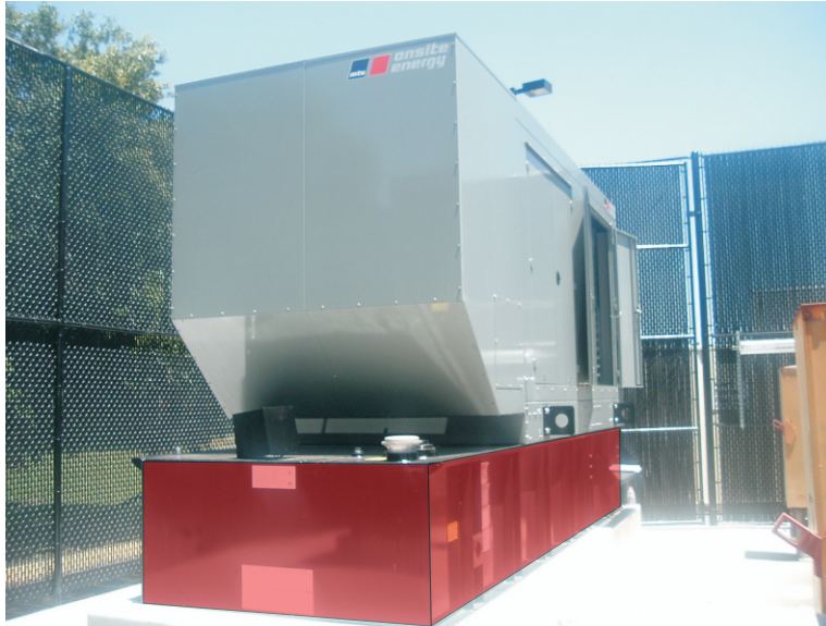
(a) Mechanical Equipment - Screened underside to prevent storage below equipment.
