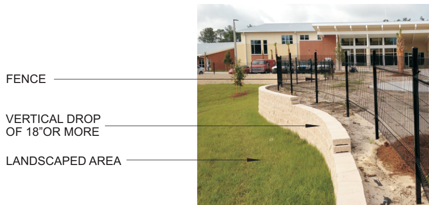
(b) Maintain protection for vertical drops
