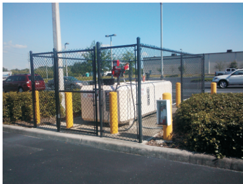
(d) Required fenced equipment - gas fueling tank
