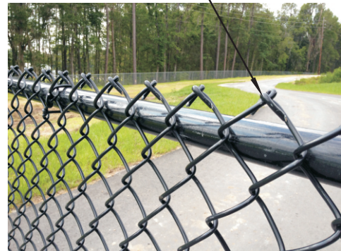
(h) Chain-link fence with turned over barb
