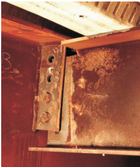
(c) Material Hazard - Damaged steel beam connection
