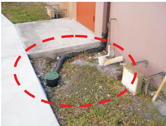
(b) Hazardous Site Conditions - Washouts around Buildings
