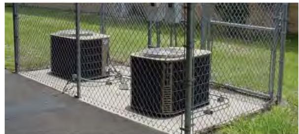
Example fencing for exposed mechanical equipment located at ground level
