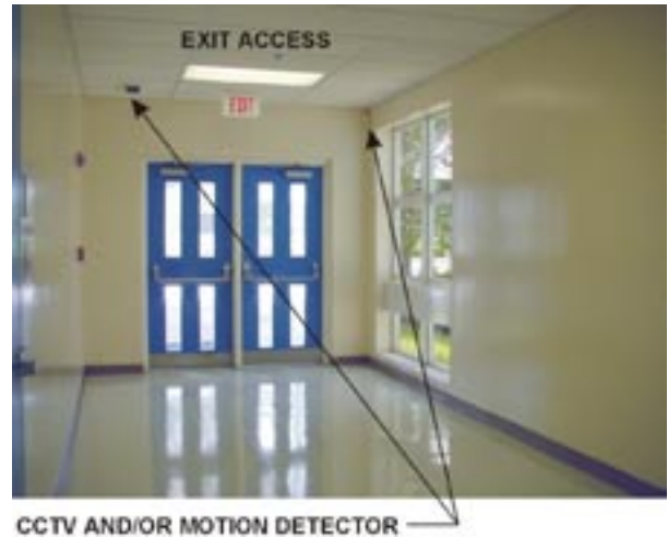
Figure 2.3.3 Secure Exit Access
