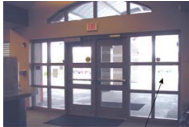
UTILIZE EXTENSIVE GLAZING AT MAIN ENTRY TO ENHANCE VISUAL SURVEILLANCE TO PARKING LOTS AND PEDESTRIAN ROUTES
