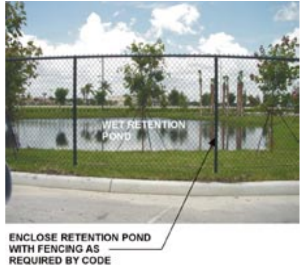
Figure 1.8.1 Fenced Retention Pond with Landscape Features
