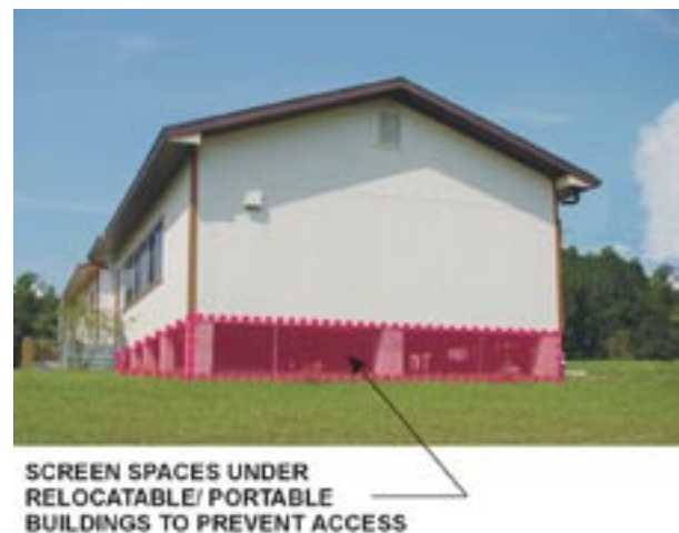
Figure 2.5.2 Example Relocatable/Portable Building
