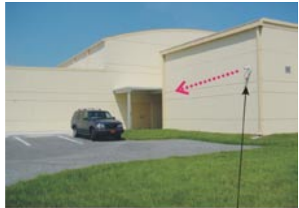
ELECTRONIC SURVEILLANCE SYSTEM STRATEGICALLY PLACED TO MONITOR BLIND CORNER AT PERIMETER OF SCHOOL BUILDING
