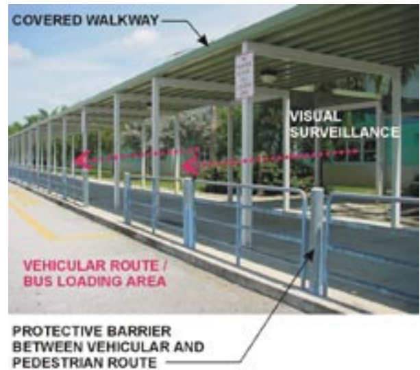
Figure 1.2.3 Bus Loading Area
