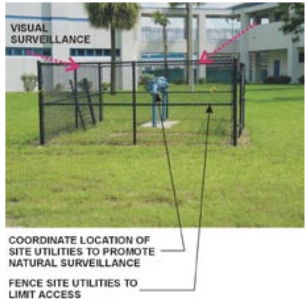
Figure 1.9.1 Secure Site Utilities and Limit Access
