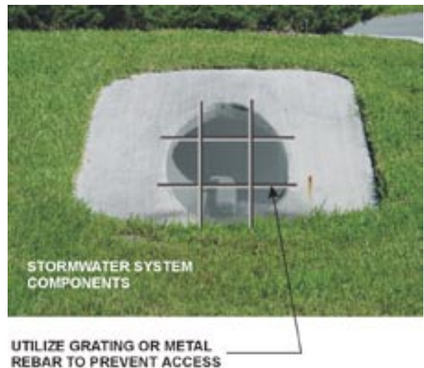
Figure 1.8.2 Prevent Access to Stormwater Structures
